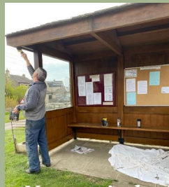
New noticeboard added & Bus Shelter painted
